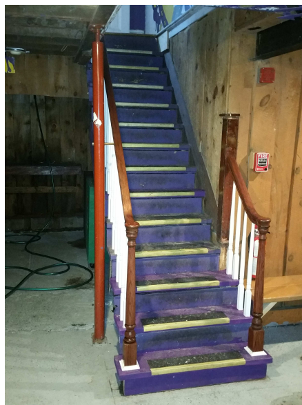
Above: New stair hand rail and balusters were installed going to the basement
